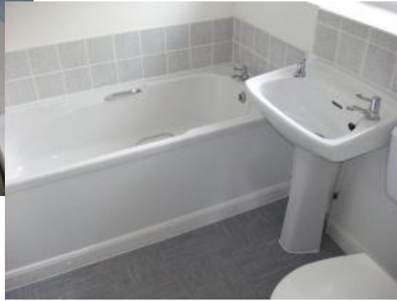
Bathroom before (downstairs off kitchen) and after (re-located upstairs)
